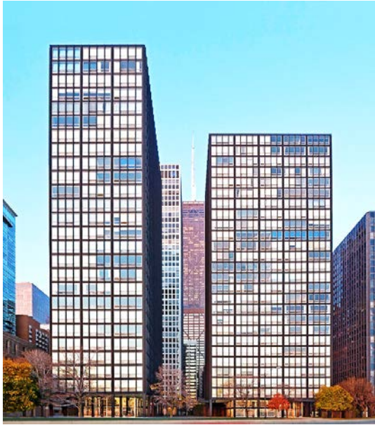
Lake Shore Drive, Chicago. Mies van der Rohe (1951)
